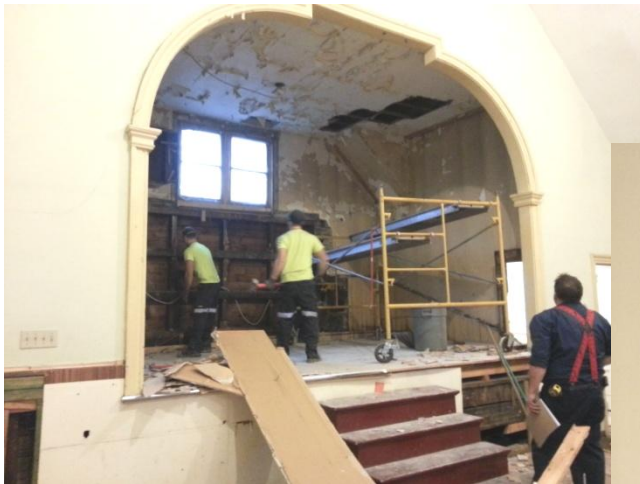
Workers dismantle the old small stage and storage area in December 2012.
