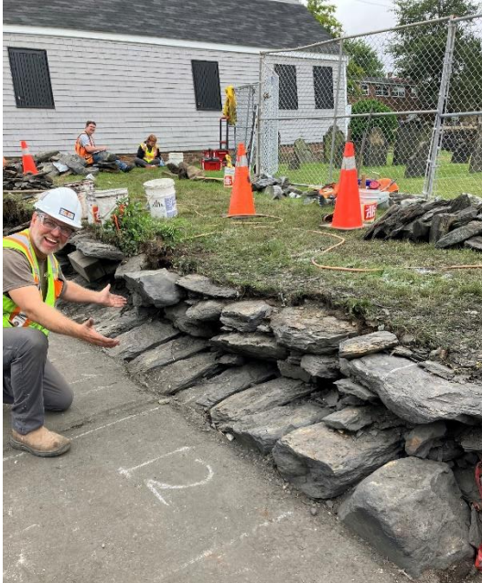
The Gerrish Street wall being dismantled.
