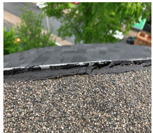
The platform on which the cupola of the Round Church sits
