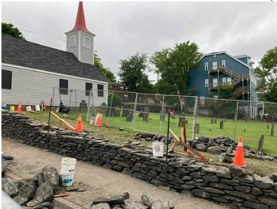
The Gerrish Street wall being rebuilt
