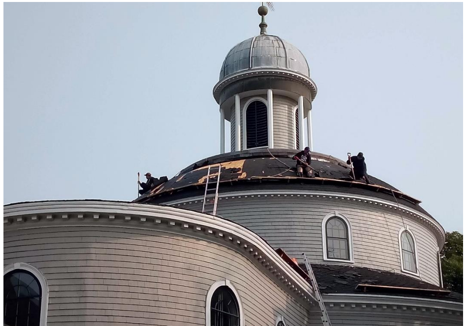
The Round Church receiving its new roof
